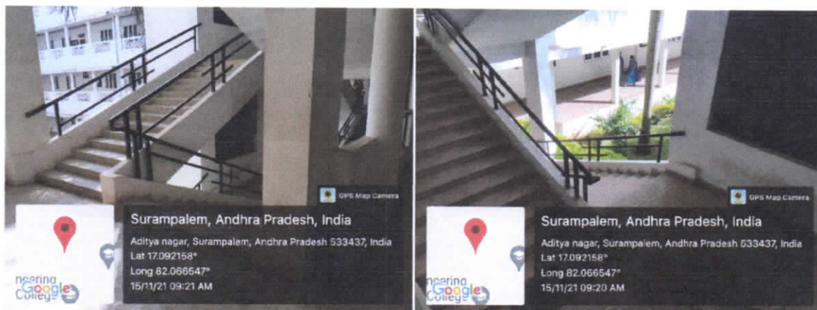
Hand Railed Stair Case
